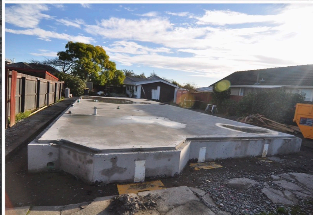
The only releveable foundation that does not require internal jacking points.
